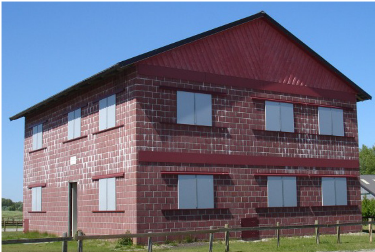
Figure F-1: Picture of an Urban Structure.
